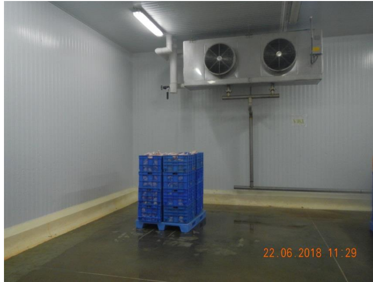
Carcass storage in chillers
