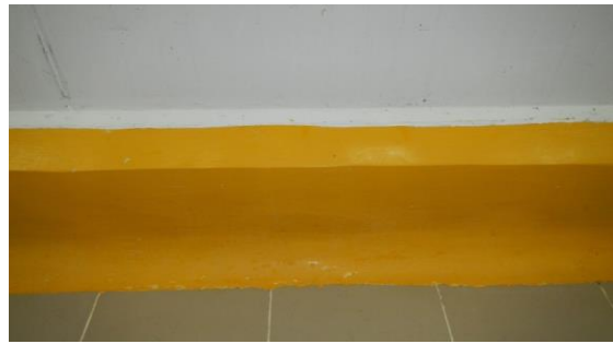
Coving between floor & wall
