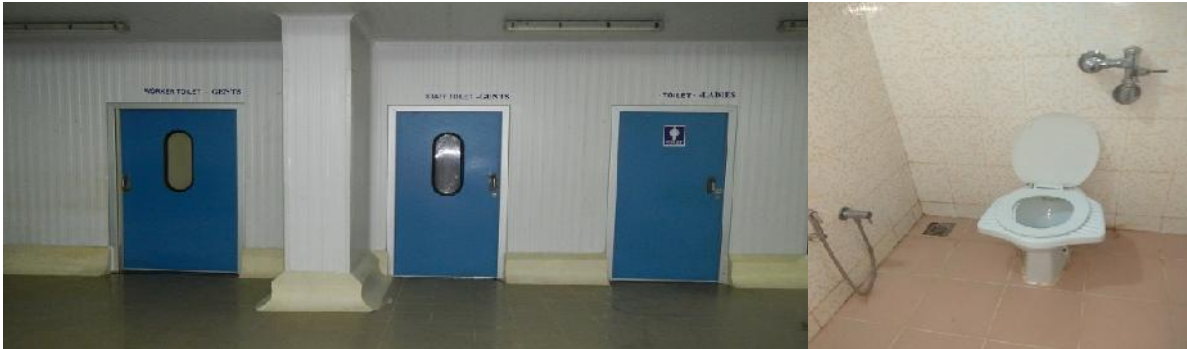
Gender Specific Toilets
