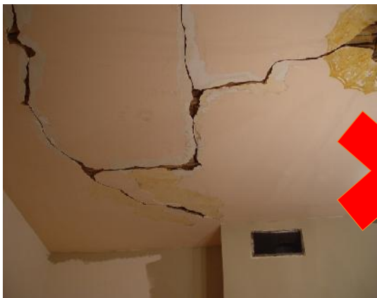
Wall and ceilings with crevices and mold growth
